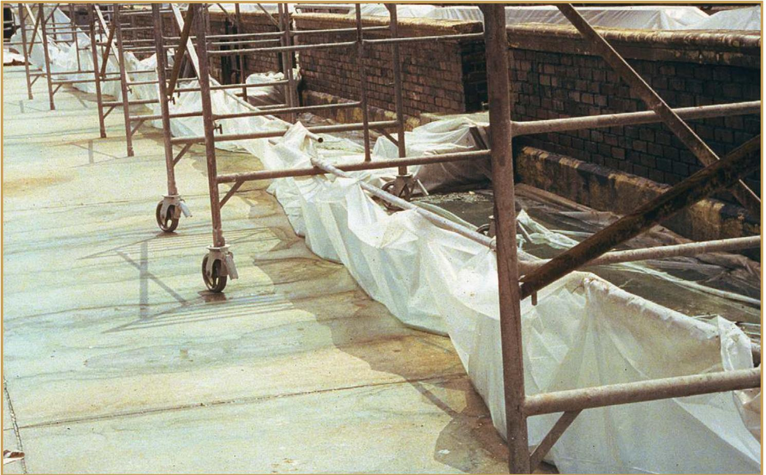
*Scaffolding holds up the back end of a plastic sheeting dam to collect paint stripping runoff during paint stripping operations at Legion Field stadium in Birmingham, Ala.*
