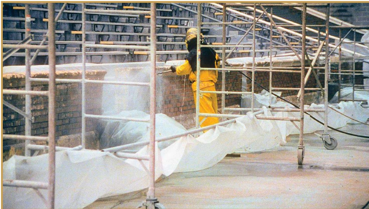
*A plastic sheeting dam catches the run-off as a technician pressure rinses dissolved paint and spent paint stripper from masonry at Legion Field stadium in Birmingham, Ala.*
