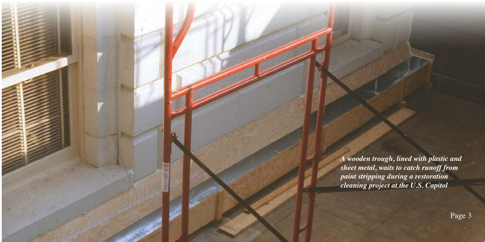
*A wooden trough, lined with plastic and sheet metal, waits to catch runoff from paint stripping during a restoration cleaning project at the U.S. Capitol*
