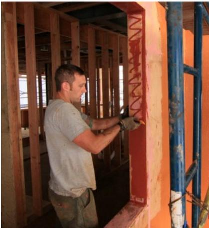
An applicator seals a rough opening against air, water and energy loss with PROSOCO R-Guard® FastFlash® fluid-applied flashing membrane. The Karuna House was designed to meet LEED® Platinum, Passive House and the Swiss Minergie ECO/P standards.
