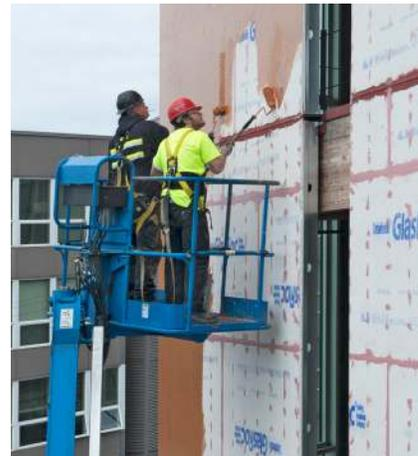
An applicator applies Cat 5® primary air & water barrier to structural walls at Seattle's Bullitt Center, the first office building to earn Living Building certification.
