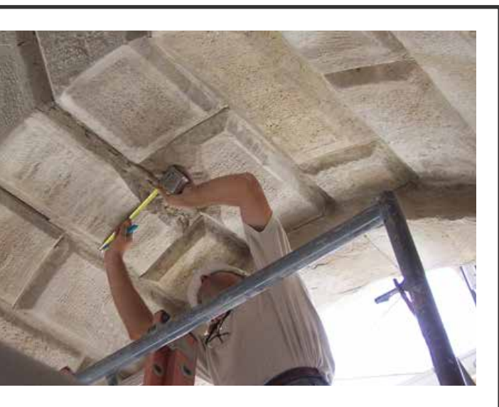
Re-anchoring terra cotta with Stitch-Ties
