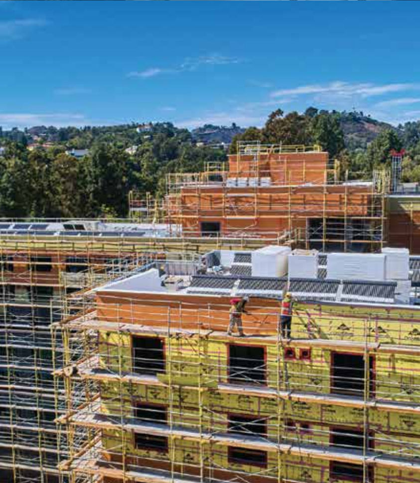
Olympic & Centennial Hall dormitories // Los Angeles CA protected with FastFlash, SureSpan EX, & Cat 5
