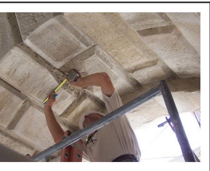
Re-anchoring terra cotta with Stitch-Ties
