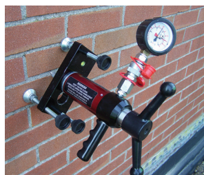
Mortar Joint Performance Test
