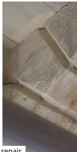
Historic limestone repair with Stitch-Ties
