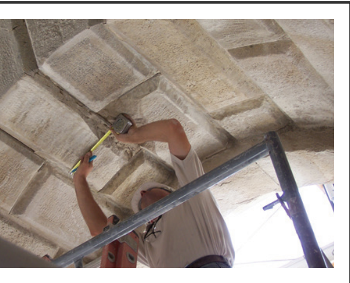
Re-anchoring terra cotta with Stitch-Ties
