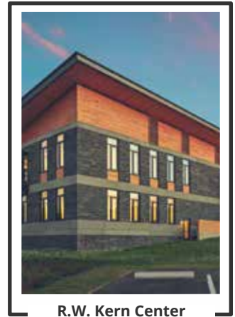
R.W. Kern Center at Hampshire College
