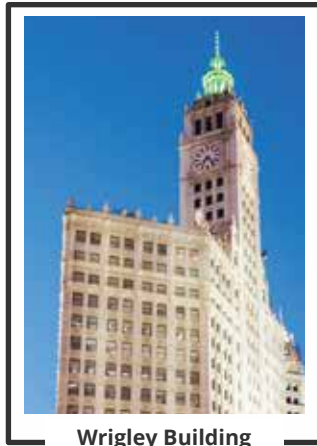
Wrigley Building Chicago, IL
