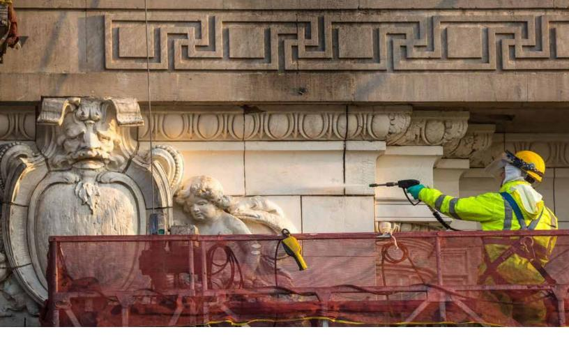
"We had the two-part chemical system (766 Limestone & Masonry Prewash and Limestone & Masonry Afterwash) as our initial recommendation, and we did at least two passes of the prewash," she said. "Some areas that were significantly soiled needed multiple passes of the prewash, and it cleaned up very nicely."
