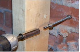
STEP 5- Thread (1) SS Lock Nut provided onto anchor shaft and position it about midway of the stud width.
