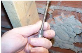
**STEP 3)** Thread shaft of SBRA anchor into the 501 Setting Tool until it bottoms in the tool.
