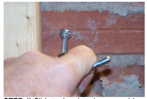
**STEP 4)** Slide tool and anchor assembly Through the drilled holes until the washer Contacts the brick face. Tighten anchor To 40-75 in-lbs torque. Remove tool.
