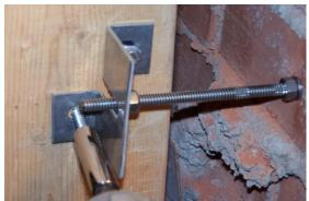
**STEP 6)** Slide on (1) SS washer provided and bracket. Secure the bracket with 2 attachment screws (provided) to the stud
