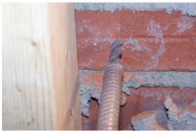
**STEP 1-** Drill ½" hole through the sheathing approximately ¼"–¾" from the stud face (parallel with mounting face)
