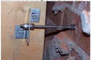
**STEP 7)** Assemble SS washer and SS lock nut to the exposed shaft and tighten until contact to the bracket is made.
