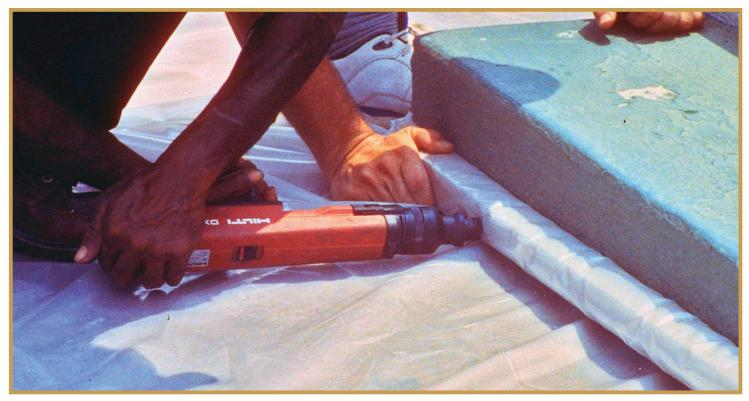
Technicians nail wood and plastic to concrete steps as they make a dam to collect runoff from an upcoming paint-stripping operation at Legion Field stadium in Brimingham, Ala.
