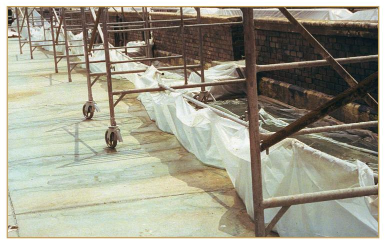
Scaffolding holds up the back end of a plastic sheeting dam to collect paint stripping runoff during paint stripping operations at Legion Field stadium in Birmingham, Ala.
