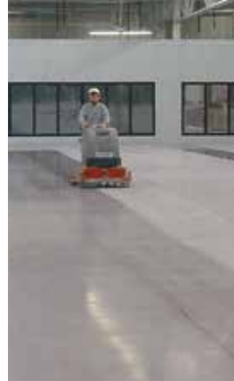
Floor cleaning with products specifically designed for interior concrete flatwork.
