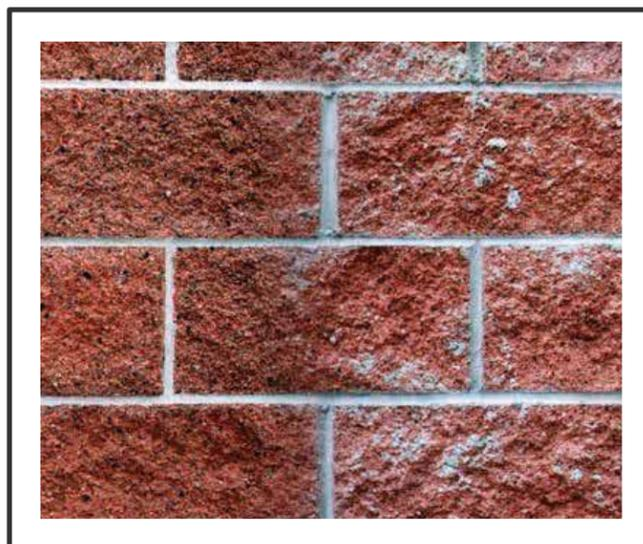
Split-faced block cleaned with Custom Masonry Cleaner
