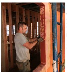
An applicator seals a rough opening against air, water and energy loss with PROSOCO R-Guard® FastFlash® fluidapplied flashing membrane. The Karuna House was designed to meet LEED® Platinum, Passive House and the Swiss Minergie ECO/P standards.
