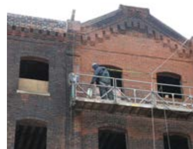
Carbon staining on brick
