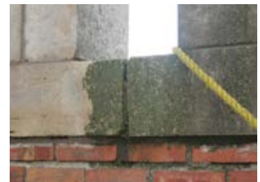
Biological staining on limestone at the Douglas County Courthouse in Lawrence, Kan.
