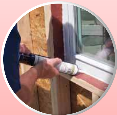
R-GUARD Air Dam® interior sealant is applied as part of the FastFlash® system for simple waterproof window installation.
