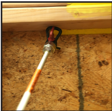
Spray application with tip guard.
