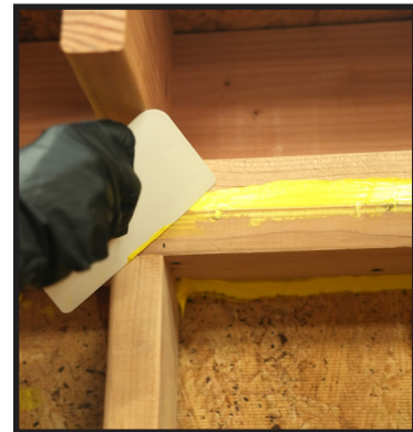
Tooling is only required at the top plate for a flat drywall installation surface.
