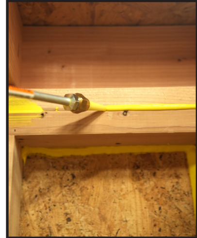
Spray application with caulk nozzle.
