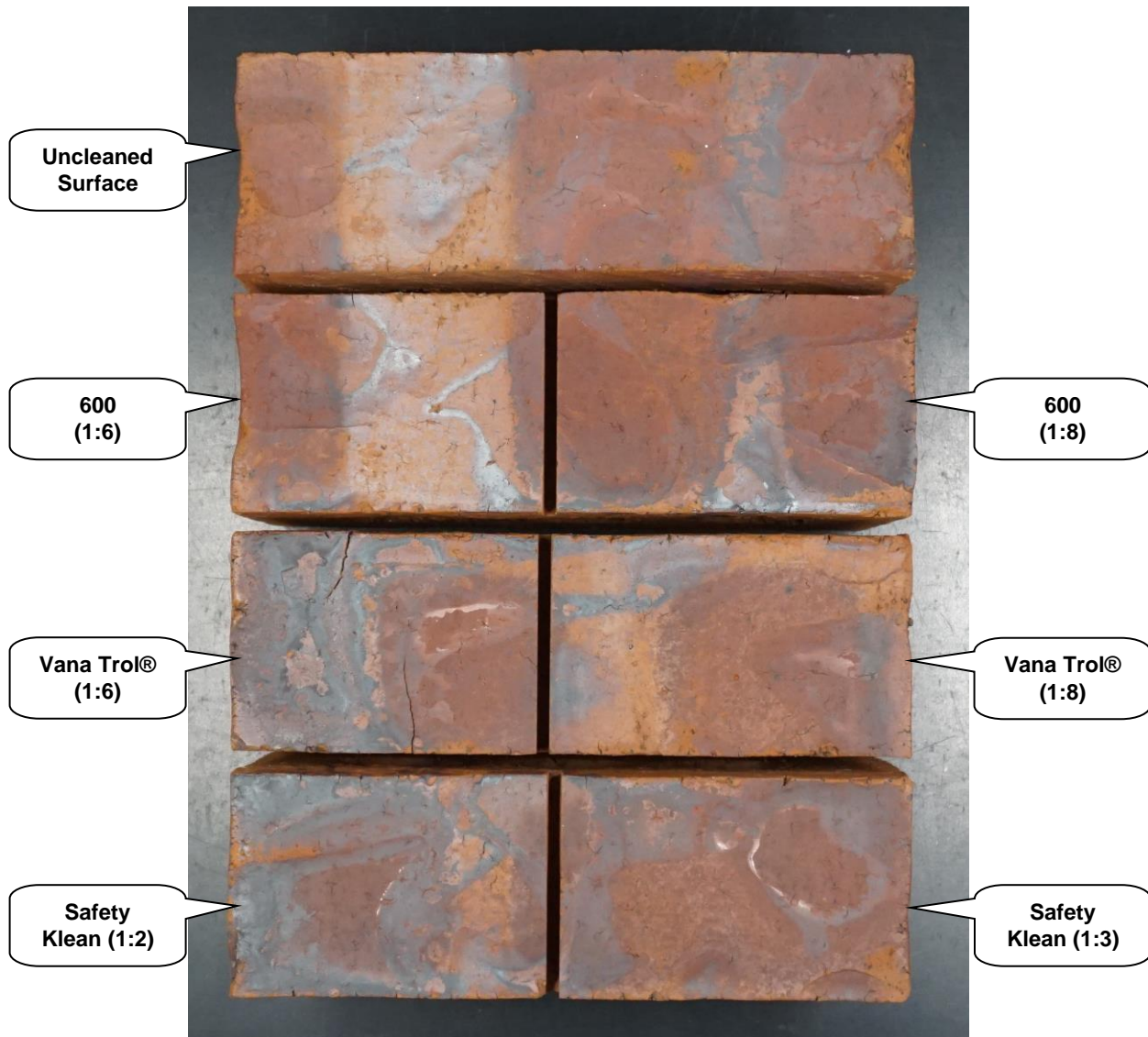
"Sheffield – Smooth" Brick After Cleaning
