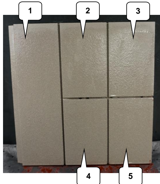
“409” Terracotta Panel Immediately After Water Rinse
