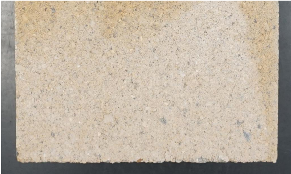
“Caliza” RockCast Smooth Masonry Veneer Before Cleaning
