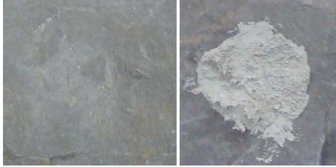
“Cajun”; 7 Day Cleaning; Type S Mortar
