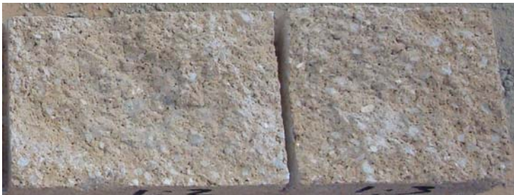
Sure Klean® Concrete Brick Cleaner (1:2)
