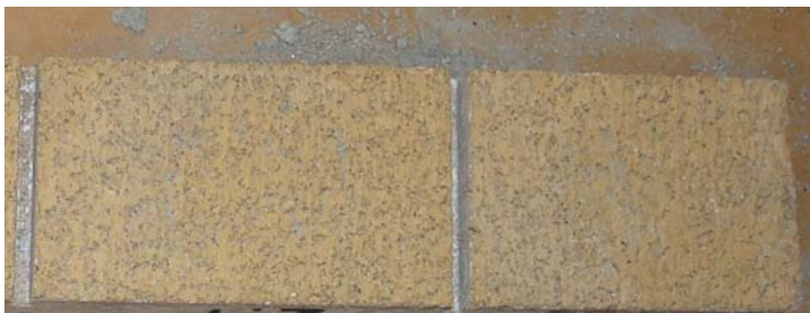
Sure Klean® Concrete Brick Cleaner (1:2)
