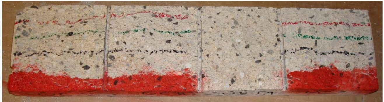
“Ivory” Split Face CMU; Before Graffiti Removal
