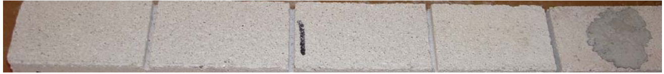
“Marble White” Smooth-Face CMU; 3 Day Cleaning
