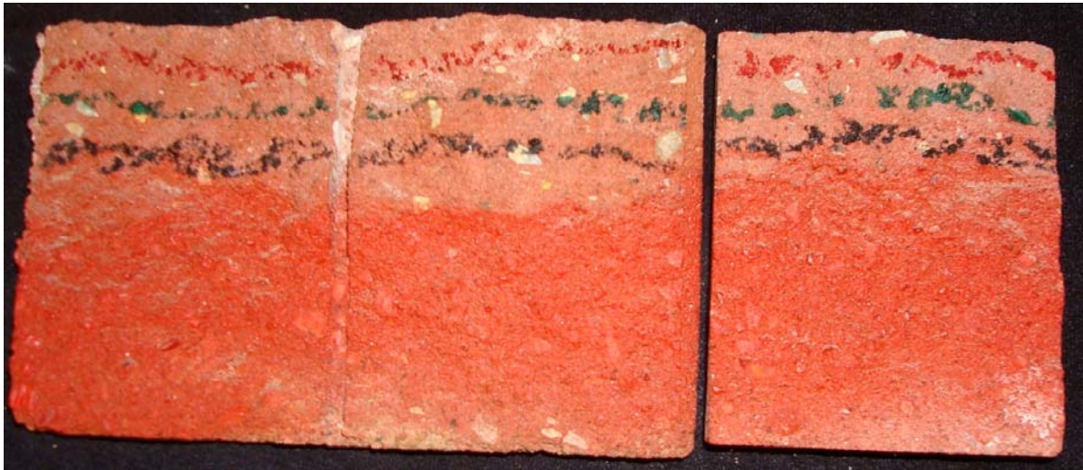
“Brick Rose” Split Face CMU; Before Graffiti Removal
