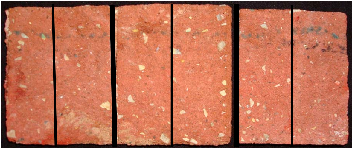
“Brick Rose” Split Face CMU; After Graffiti Removal
