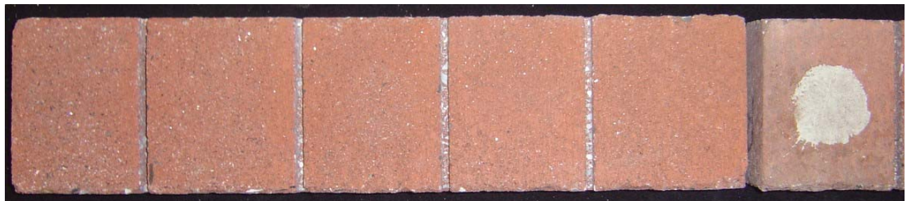
“RLB” Concrete Brick; 14 Day Cleaning
