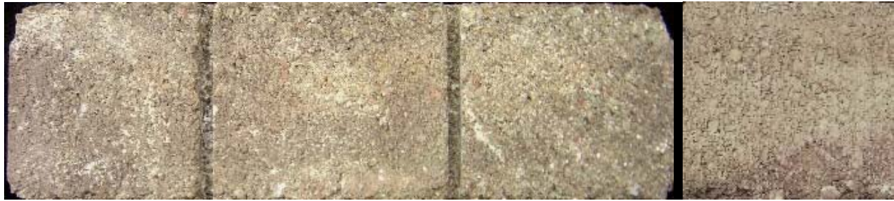
Sure Klean® Concrete Brick Cleaner (1:2)
