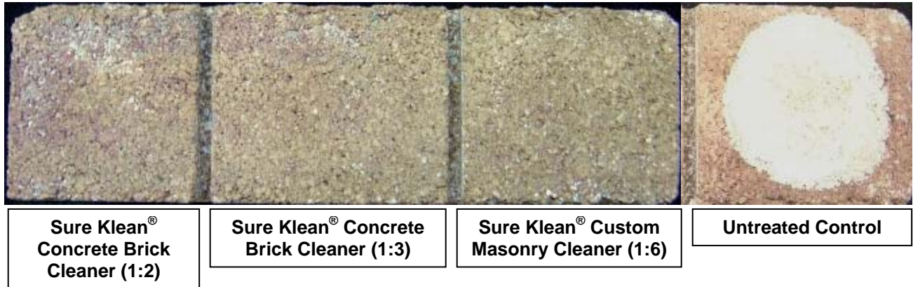
“Niota” Concrete Brick; 7 Day Cleaning
