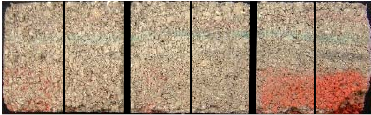
“Leatherwood” Concrete Brick; After Graffiti Removal
