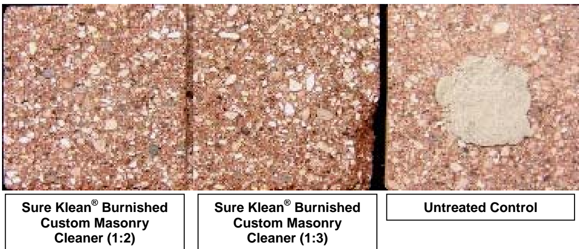
“Old Red” Ground-face CMU; 14 Day Cleaning
