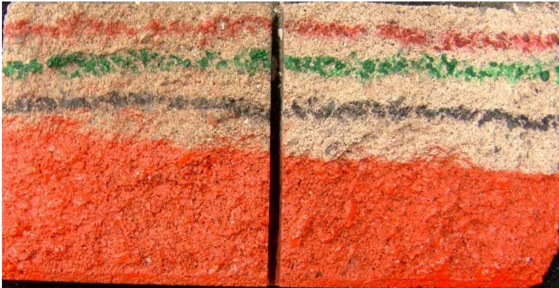
“Sahara” Split-face CMU; Before Graffiti Removal
