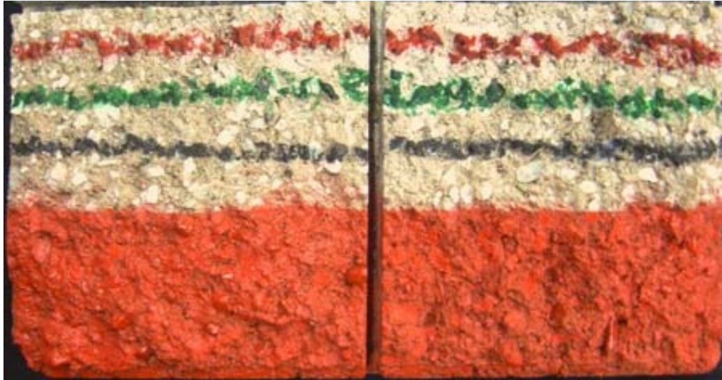
“345” Split-face CMU; Before Graffiti Removal
