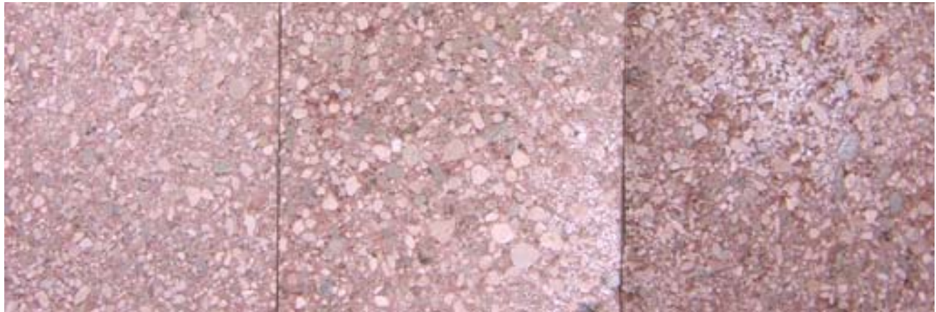
"364" Ground-face CMU; Treatments Applied
