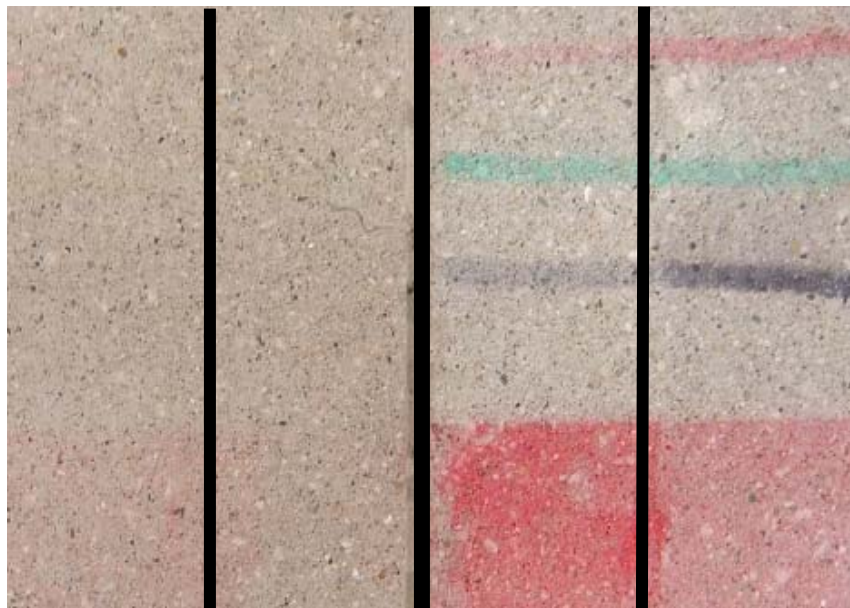
“WC1090”; After Graffiti Removal
