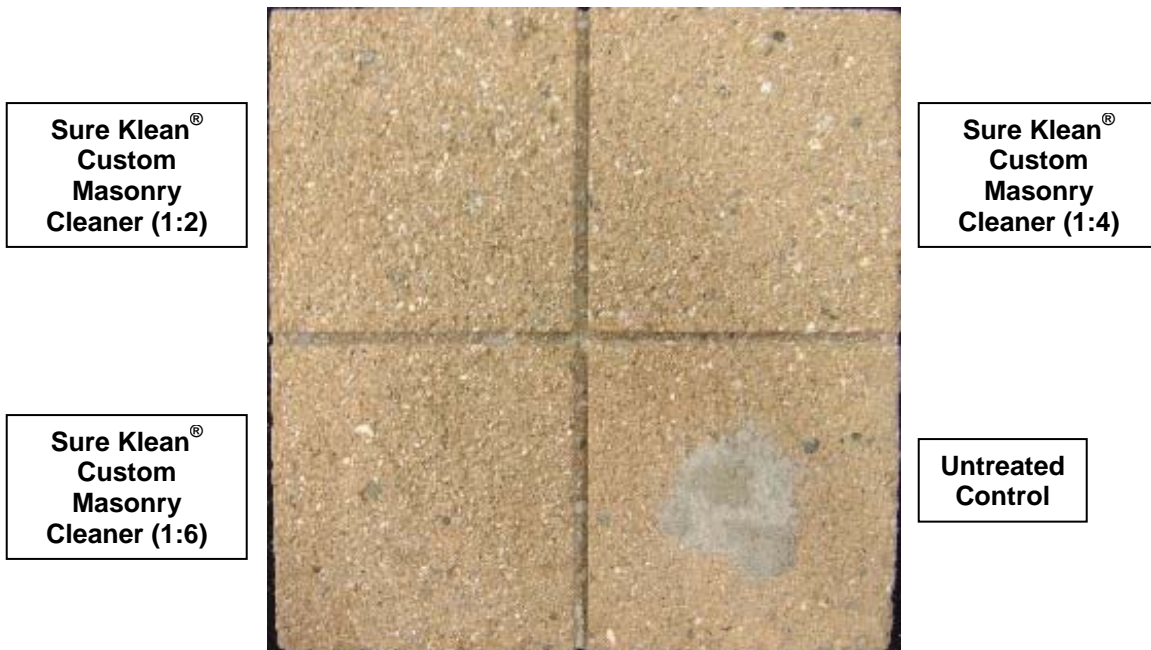
“70D” “Steel Shot Blasted” CMU; 7 Day Cleaning
