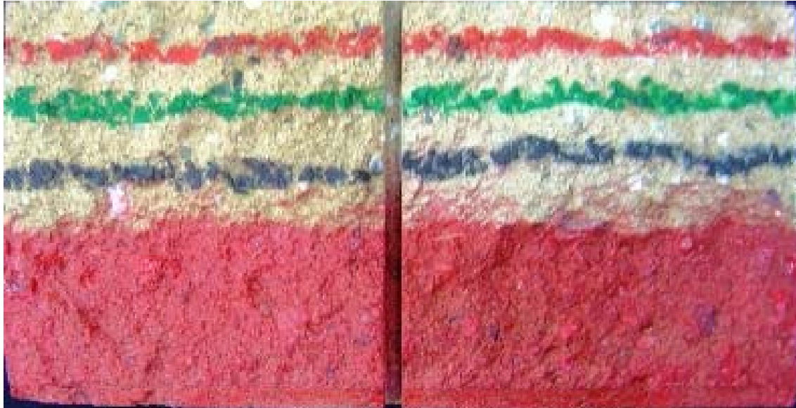
“87” Split-face CMU; Before Graffiti Removal
