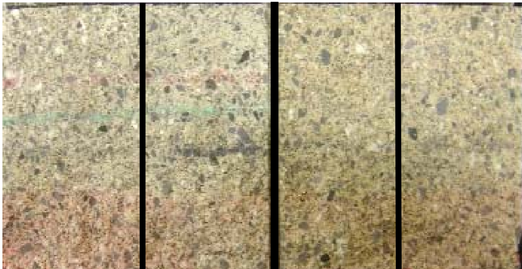
“Buff LW” Split-face CMU; After Graffiti Removal
