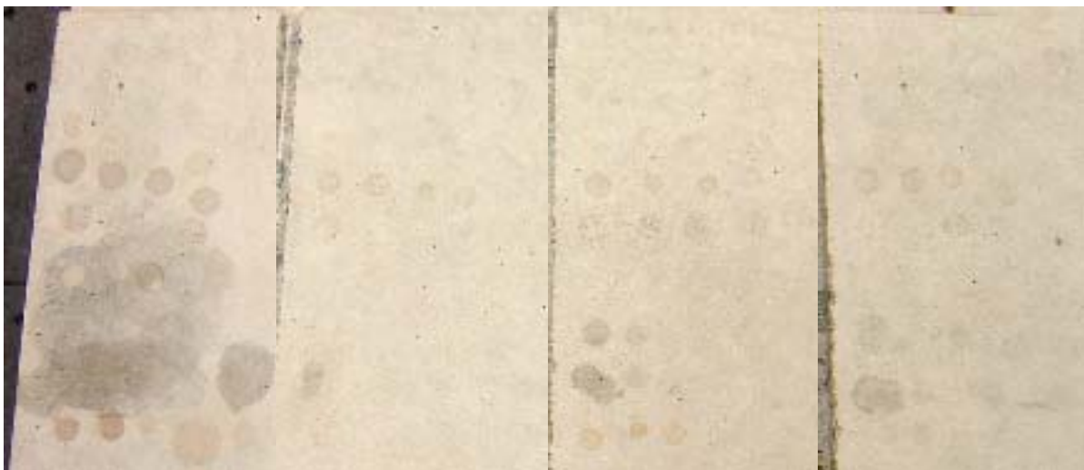
“Granada White” Wall Cap; Stains Removed
