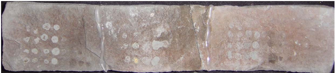
“Slate”- Stains Removed
