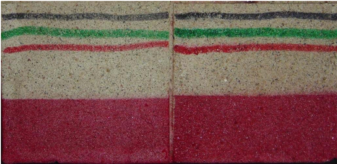
“9-3-02A” Dry-Tamp Cast Stone Before Graffiti Removal
