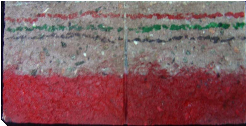
“6032 (Brown)” Split-face CMU Before Graffiti Removal
