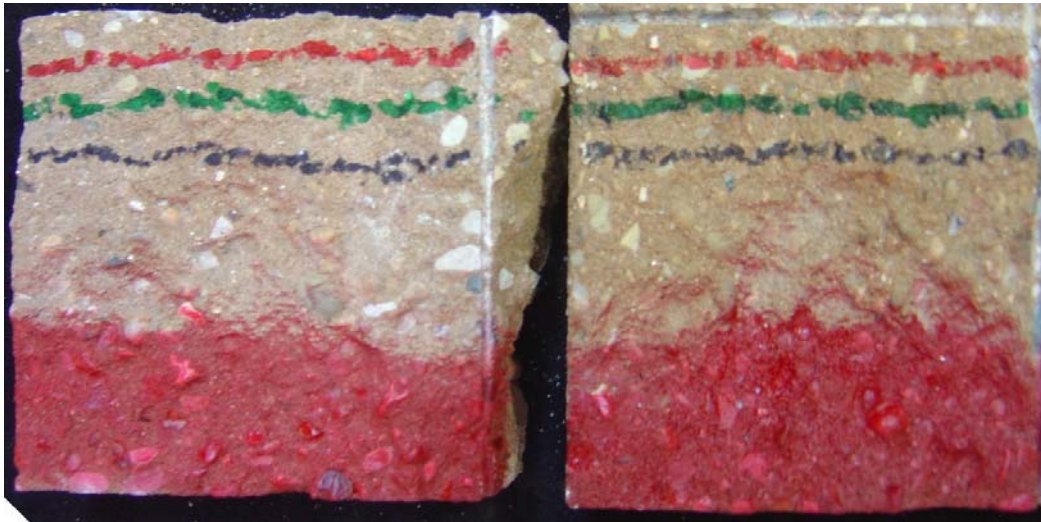
“51-042” Split-face CMU Before Graffiti Removal
