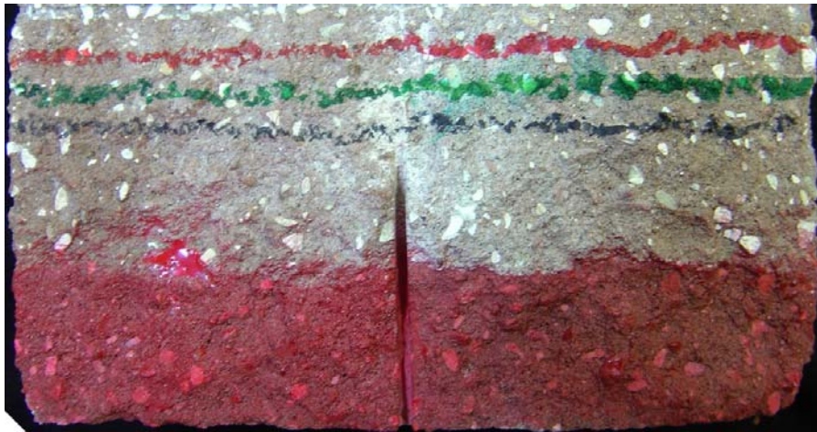
“Sienna” (6) Split-face CMU Before Graffiti Removal
