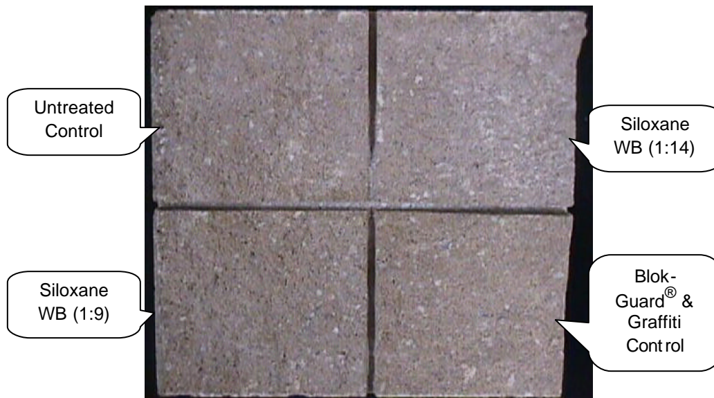
“Sunset” split-face CMU after water repellency treatment
