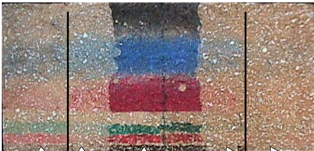
Photo of split-face CMU “#55” after cleaning:
