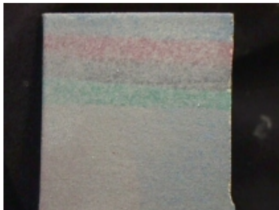
Picture 2.3 – Graffiti has been about 70% removed from the untreated surface, leaving mostly the permanent marker residual graffiti behind.
