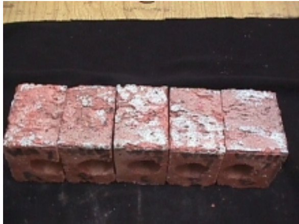
Wellsley before cleaning
