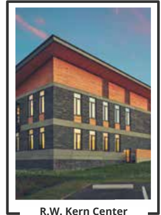
R.W. Kern Center at Hampshire College
