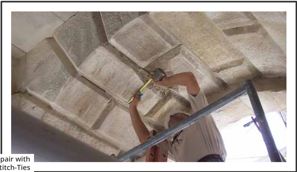
Re-anchoring terra cotta with CTP Stitch-Ties
