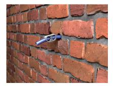
11. After a few minutes, fasten the clamp before turning off the compressor. It is advisable to remove the hose from the threaded tube 2-3 hours after installation. Wash any excess grout off with clean water, then fill the holes with SureFill flexible pointing mortar and colour match the masonry with Surestain.
