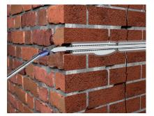
9. When the sock has been fully inflated, milk grout gently runs from the anchor indicating that it's full.
