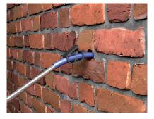
Once ready to fill, slip a clamp over the exposed hose, then push fit the steel pipe into the open end. Switch on the compressor and proceed with pumping.
