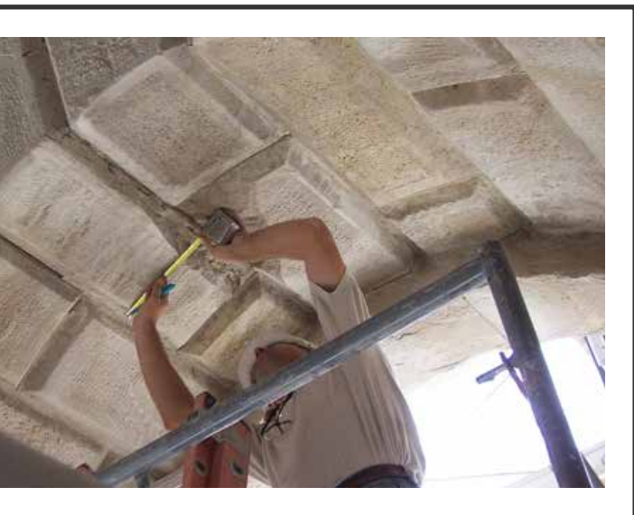
Re-anchoring terra cotta with Stitch-Ties
