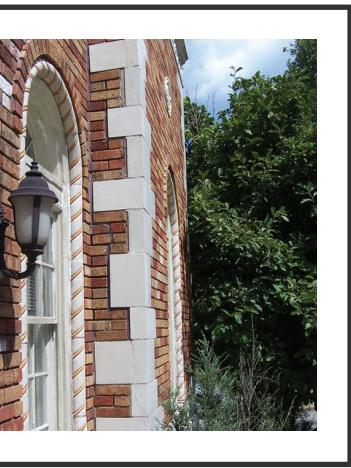
Re-anchoring to metal stud with Stitch-Ties
